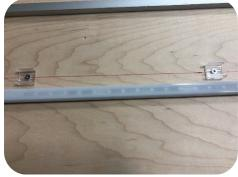
Mounting clips centered on guide line. Space clips as needed.
