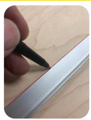
Use a straight edge, mark a line for the center point of the encapsulated line bar.
